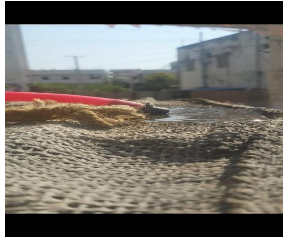
Figure.9 showing Pump flushing water making mat wet.
