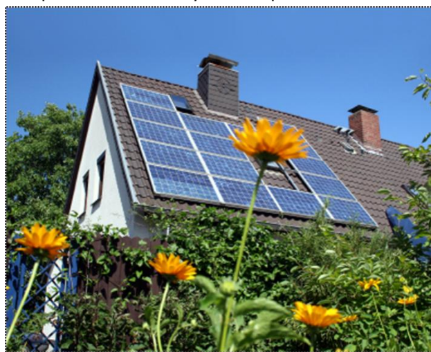
Figure 1: Solar panels on the roof
