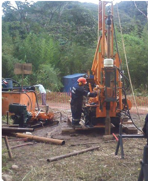
Figure 2. Piezometer Drilling 01 (Pz-01)
