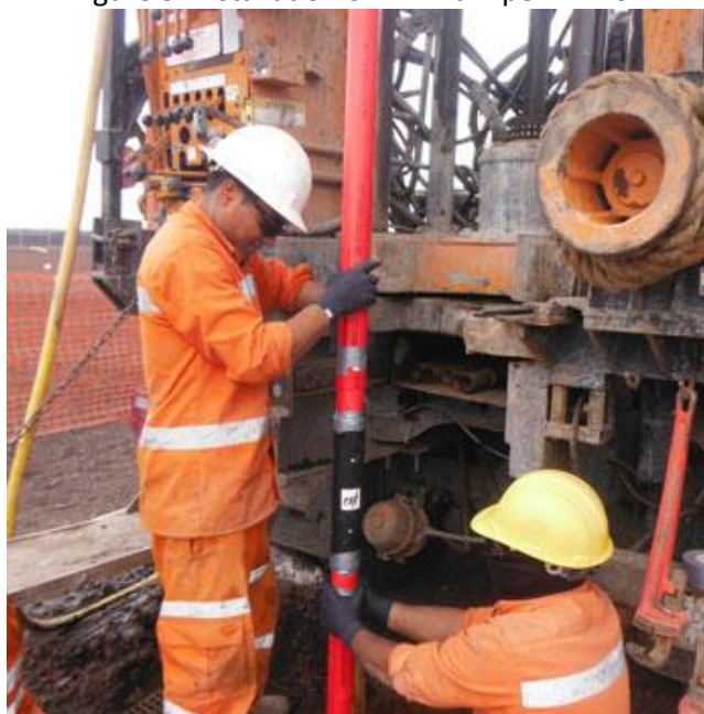
Figure 3. Installation of 2 Blind Pipe in Pz-01.
