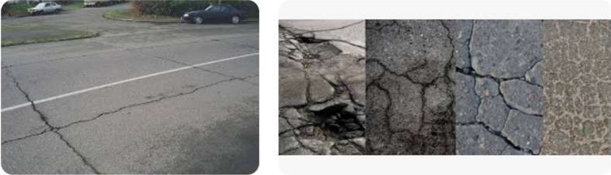
Fig:2 Cracking and Joint Damage
