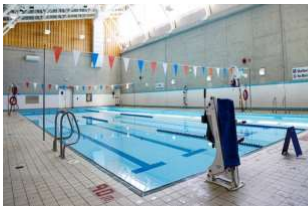
FIGURE 1. Indoor swimming pool (ISWP)
