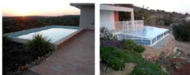
FIGURE 32. Views of the NC and 2C swimming pools are shown from left to right 48 .
