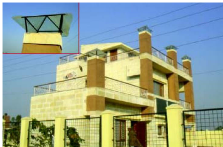
Fig 8. Picture showing building integrated solar chimney in Sudha and Atam Kumar's residence at New Delhi for effective ventilation, especially during the humid season.
