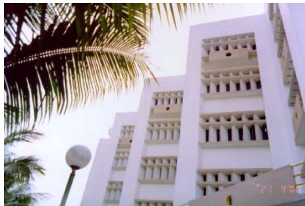
Fig 7. The office building for the West Bengal Pollution Control Board is a landmark of energy and resource-conscious architecture in this region. Efficient planning and carefully designed shading devices, fenestration design and efficient lighting design have brought about 40% energy savings over a conventional building of similar size and function. This picture shows the east facade with inclined louvers to cut off solar gains.
