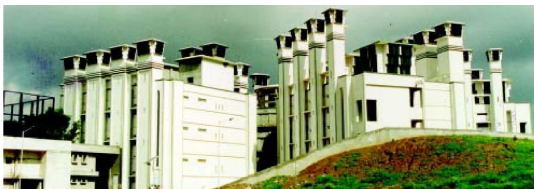
Figure 12. Passive downdraught cooling has been successfully used at Torrent Research Centre, Ahmedabad. The wind catchers for the system are the predominant architectural elements in this building.
