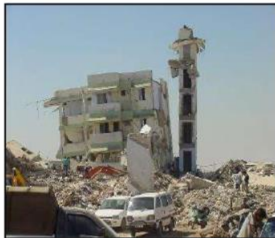
Figure 1- Apartment collapse in 2001 Bhuj earthquake with separation of the lift shaft
