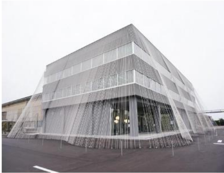
Figure 3- Structure made with carbon fibremateria
