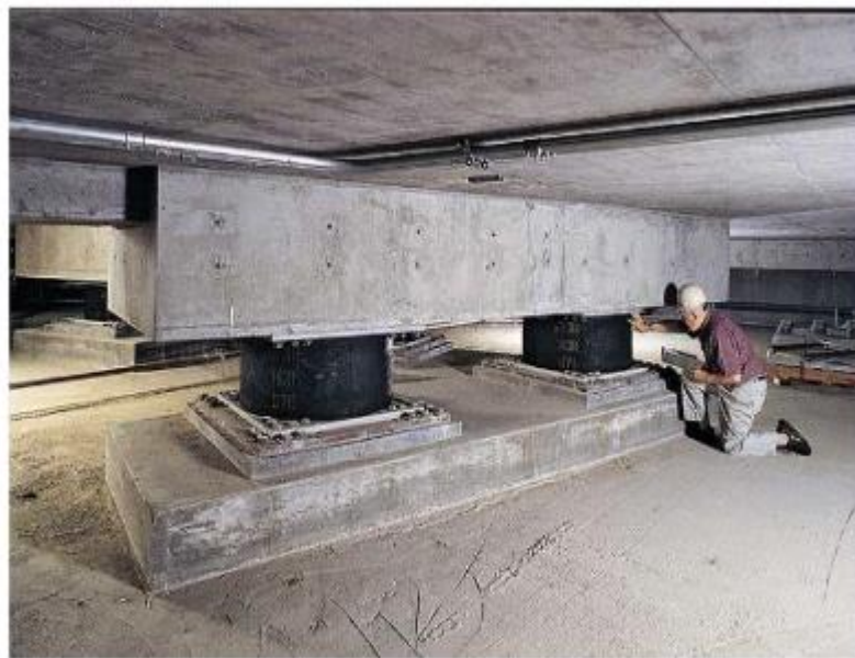
Figure 2- Base isolators
